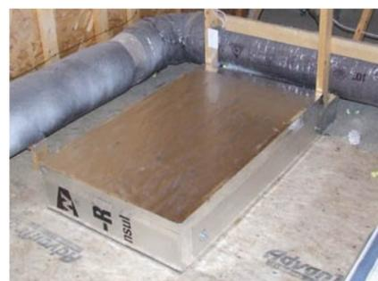
Insulated attic hatch and insulated ducts
