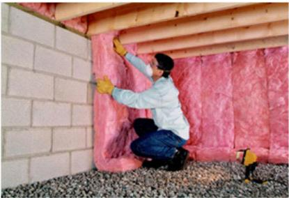
An example of proper installation (no vent)
